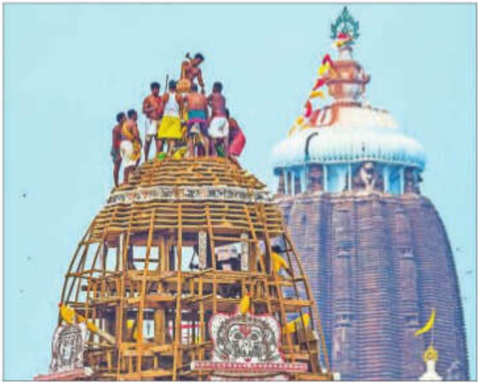
Workers fix the dome and give final touches ahead of the Rath Yatra festival near Jagannath Temple in Puri. PTI
